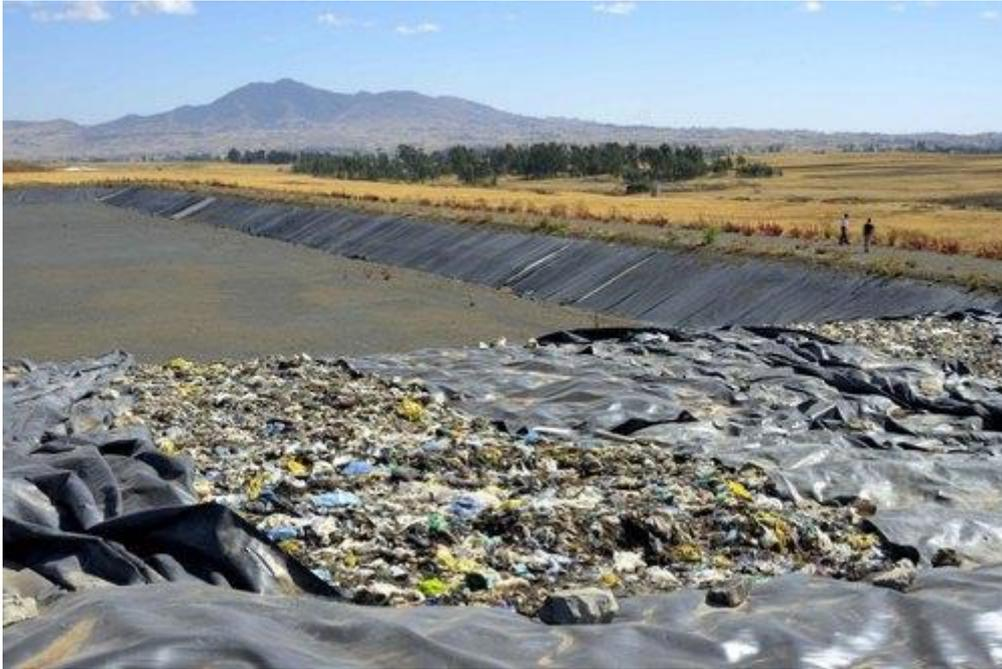
**Gambar 4** *High Density Polyethylene Geo-membrane* [10].
