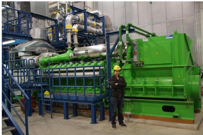
**Gambar 5 Gas Engine for Electric Power Generation [11].**
