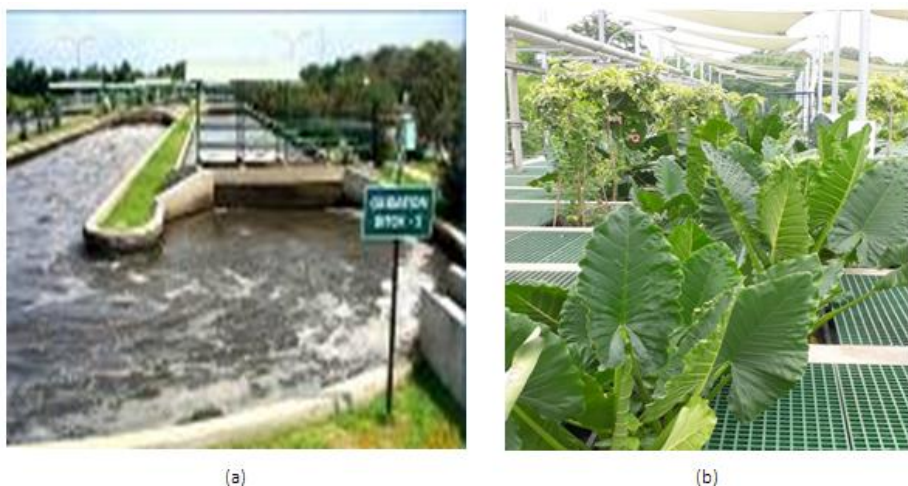
Fig 2. Appearance of WWTP using conventional oxidation ditch (a) and WWTP after with Organica-FCR technology (b) source: Documentation of Jababeka
