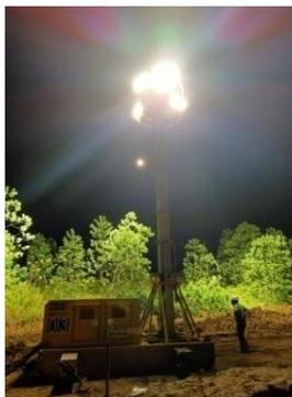
Gambar 2. *Tower lamp* 12 meter terpasang lampu LED NL500D.
