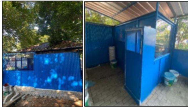
Figure 4 : Maggot Cultivate Facility Area
